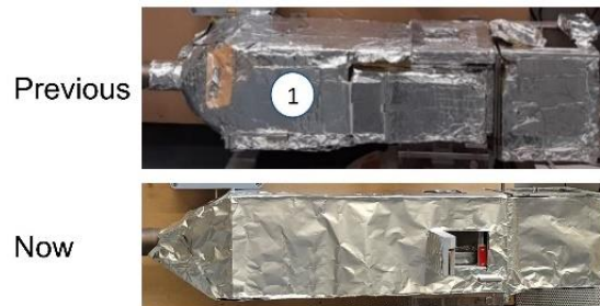
Figure 4: The external insulation material of the film dryer was replaced from fire-resistant cotton to calcium silicate boards.
